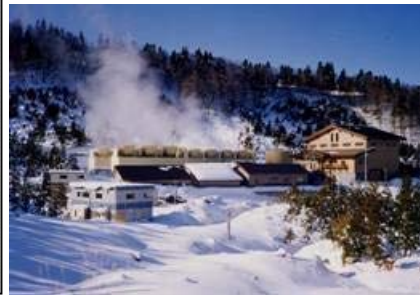
[上の岱地熱発電所]
